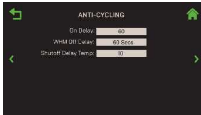
Figure 4.3.4.2: Operating Controls: Anti-Cycling Control Screen – Innovation
