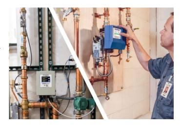
The IntelliStation digital water mixing system delivers mixed hot water throughout a hot water recirculation loop in commercial and institutional facilities. Intelligent control of the water recirculation loop ensures safe, precise, and consistent water temperatures, supports energy conservation, and reduces energy costs.
