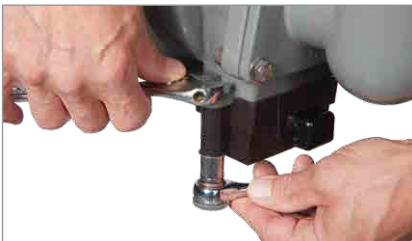
3. Use the two wrenches to tighten the bolts securing the sensor to the valve.
