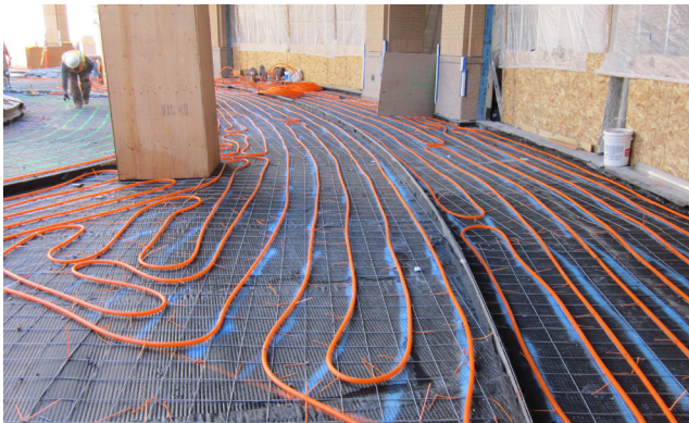
Watts Radiant® and SunTouch snow melting systems
