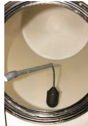
Pre Installed Float Switch
