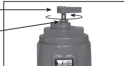
Sizes: 1 1/2" through 3" Turn knob 6-8 turns counter-clockwise
